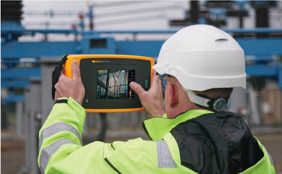
Image taken of the ii910 Precision Acoustic Imager detecting partial discharge in a high voltage application.
